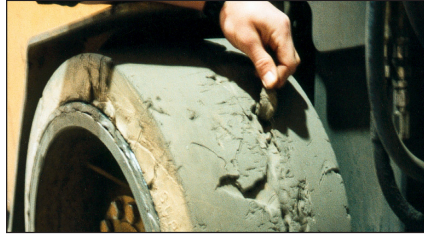
Floor defects and poorly maintained floors substantially increase material handling vehicle damage and wear, leading to increased costs and very likely an unhappy tenant.
